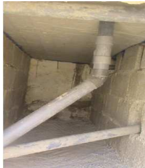
Fig. 5: Pit in construction sheltering various pipings
