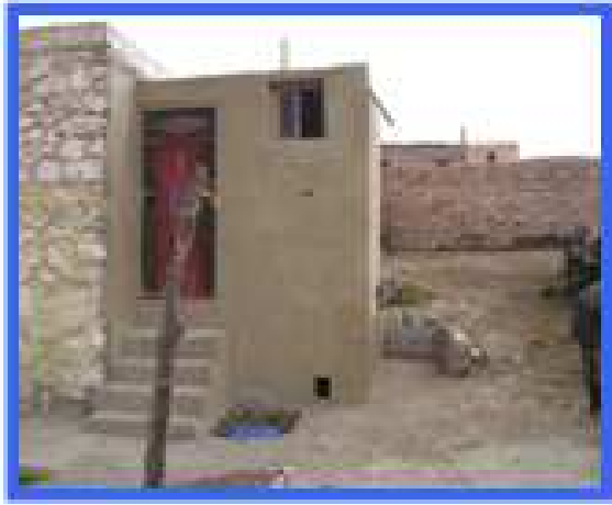
Fig. 6: UDDT built in June 2009
