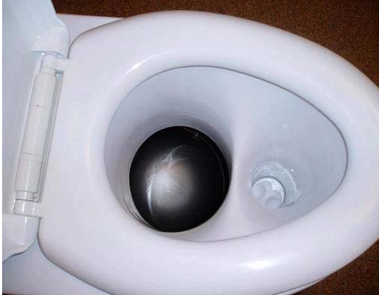
Figure 3 Urine diversion toilet and turning bowl
