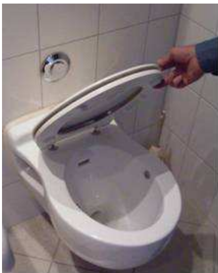
Fig. 5: Vacuum toilet (source: Otterwasser)
