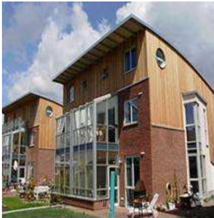
Fig. 4: Twin houses in Flintenbreite (source: Otterwasser GmbH)
