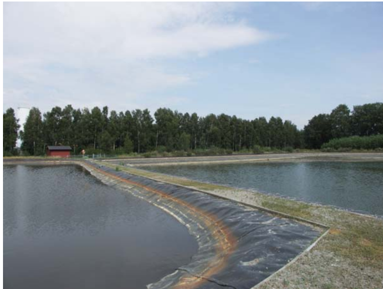
Figure 23: Storage dam for blackwater, Enköping. (source: Cecilia Toresäter, Enköping municipality)
