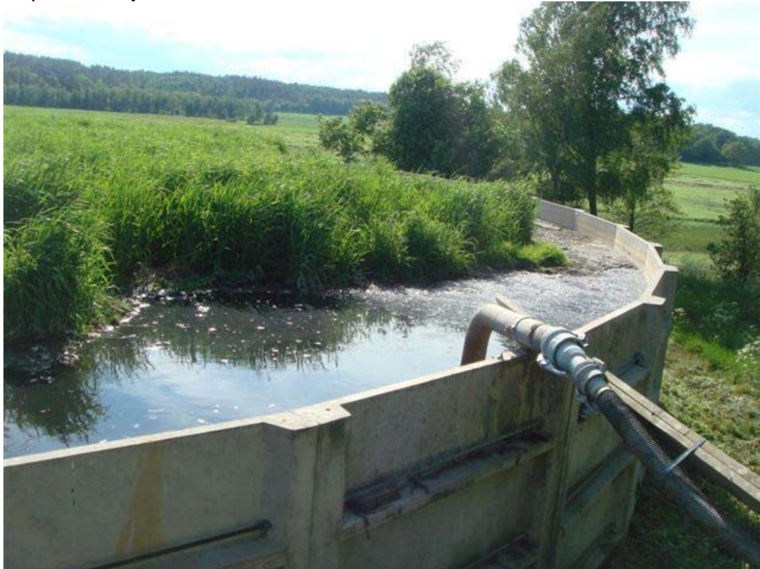
Figure 18: Emptying a tank truck into storage tank. (source: Anna Smolka, CCB Water Policy Officer)
