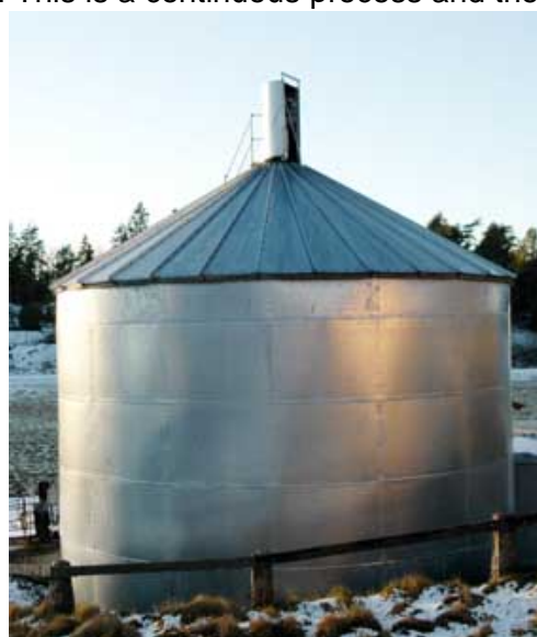
Figure 20: Digestion chamber. (source: Bosse Karp, 2006.)
