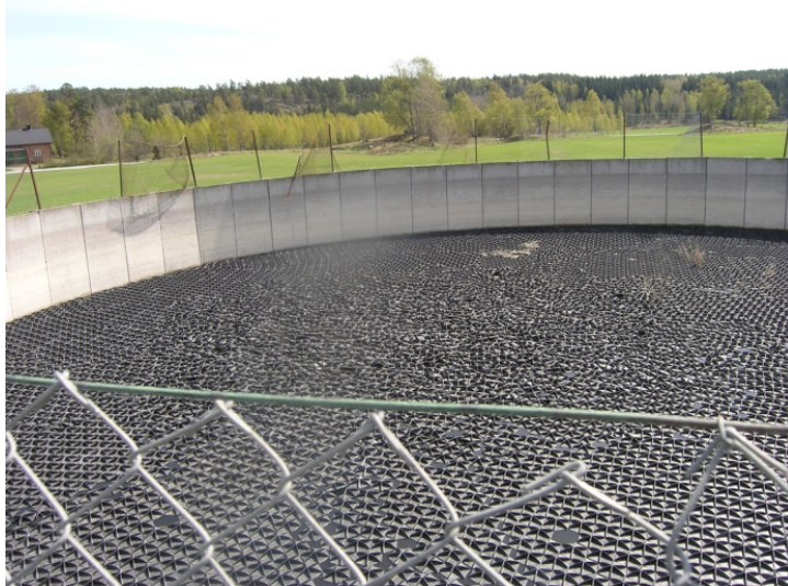
Figure 14: floating cover of storage facility (source: Ebba af Petersens)
