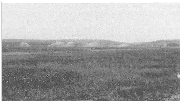
Figure 11-2. Solid set sprinklers apply tomato processing wastewater to overland flow slopes.
