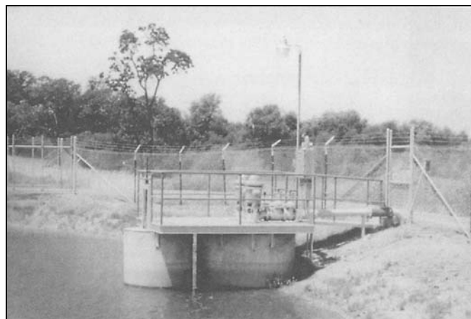
Figure 7-20. Distribution Pumps in the Side of a Storage Pond Dike.
