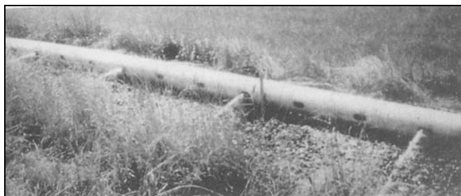
Figure 7-2. Typical Gated Pipe Distribution Unit.
