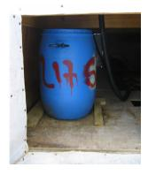
Photograph 2. 15-gallon drum with wooden guides.
