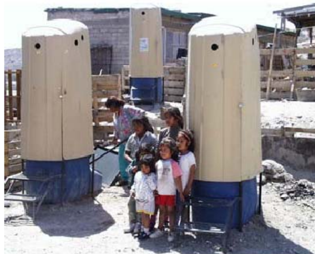
Figure 11: The SIRDO is a composting toilet that requires no water and very little space. The photo shows some units in Cuidad Juarez, Mexico.
