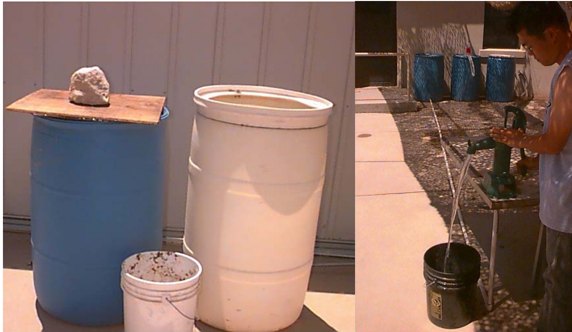
Figure 25: A typical water storage system consists of open top recycled drums. A closed system with a pumped delivery can be assembled at a relatively low cost.
