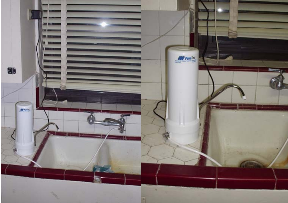
Figure 4: Here is a counter top version of a UV treatment device. It also includes a carbon block filter to improve taste.
