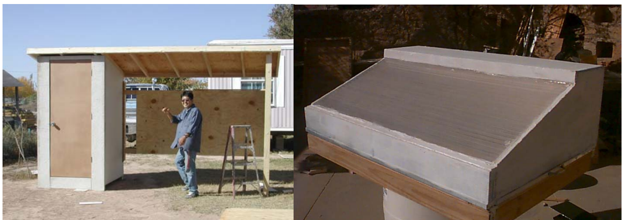
Figure 13: The collection of waste can be almost anywhere. The demonstration unit (above, left) was constructed like a pit privy but with bag collection. The pasteurizing hot box (right) is a simple, glazed and insulated box that resembles a solar cooker.
