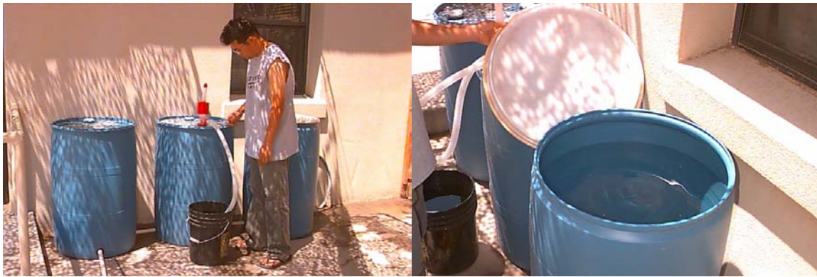
Figure 26: New or recycled drums can be connected with Uniseals and PVC pipe. A siphon pump allows the owner to draw water without contaminating the supply. One removable head drum makes it easier to fill the system.
